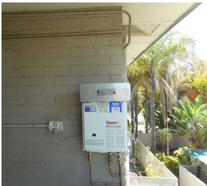
Replacement compliant water heater
