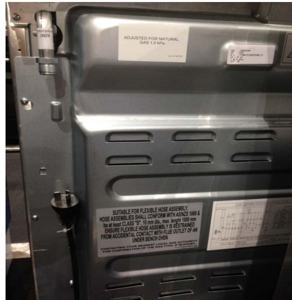
High-level connections on freestanding cookers
