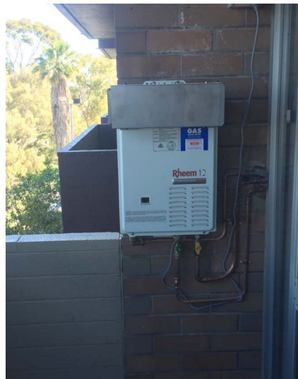
Replacement compliant water heater
