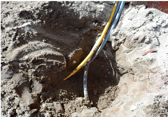
Photo 3: Minimum 600mm separation required between water services (grey pipe) and gas (yellow pipe), because there is no indicator tape or mechanical protection to the gas service.
