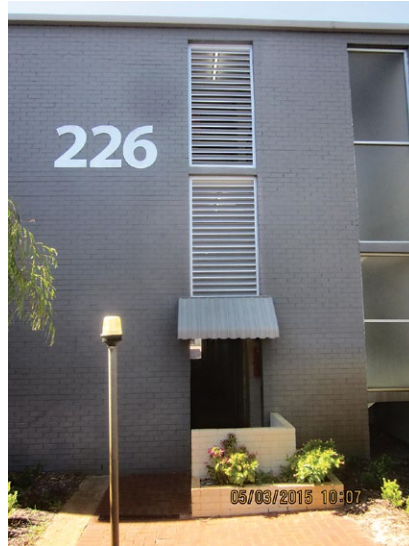
Louvered fixed vents installed
