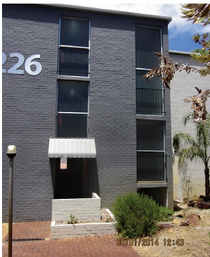
Original sealed corridors
