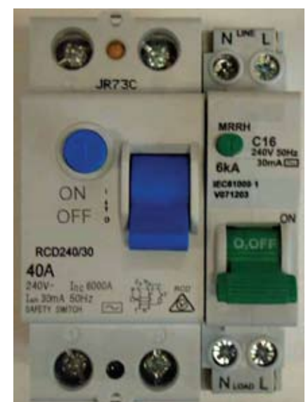
The new compact single pole DIN mounted combined RCD/ACB compared to the 2 pole conventional RCD
